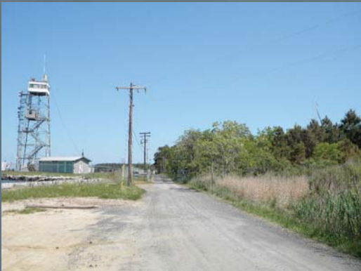
Management Area Entrance- approx. location for interpretive resources and trail head
