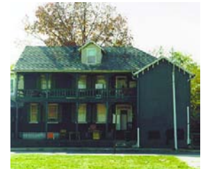
Victorian era structure along Frederick Avenue near Gwynns Falls
