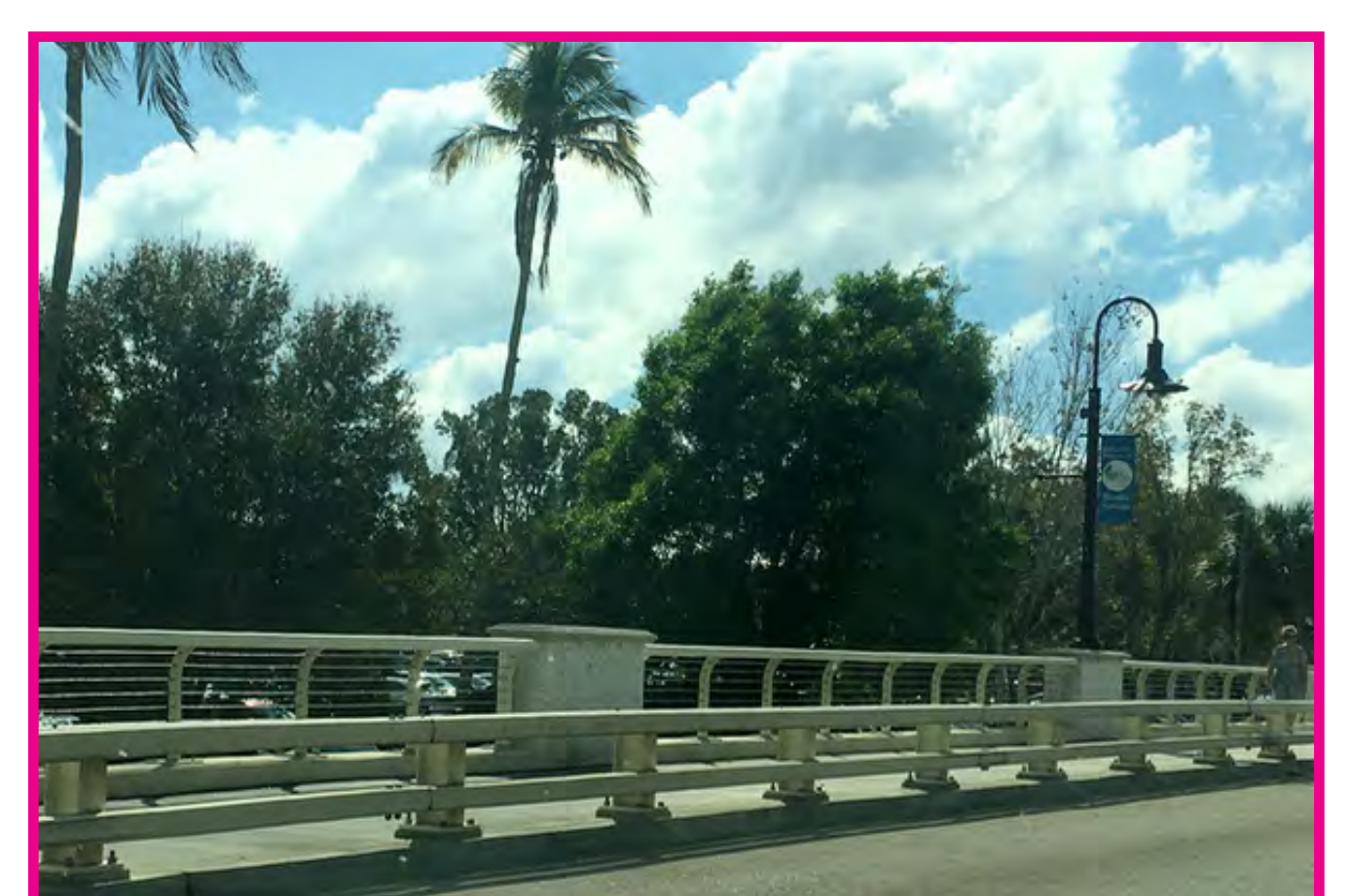
Box beam (inside) and pedestrian railing (outside)
