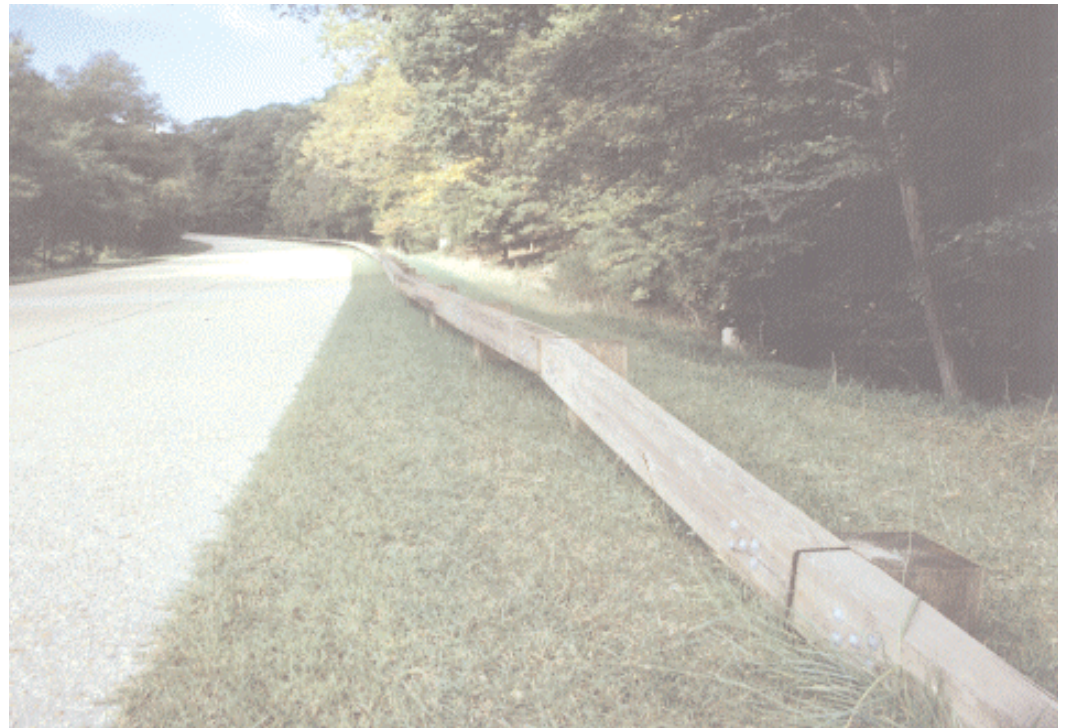
Example of steel-backed timber guardrails.
